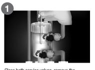
Close both service valves, remove the magnet and drain plug to drain the Magflo filter.
