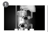
Close both service valves, remove the magnet.
