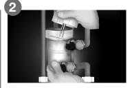
Open the lid with the spanner provided, supporting the Magflo filter with your other hand. Remove the inner filter and clean manually.
